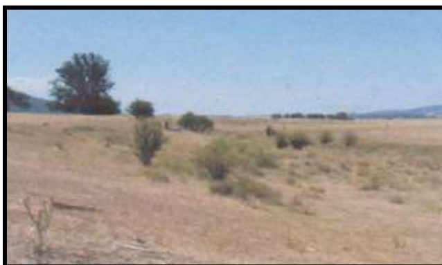
Woolshed Embankment near the Lake George Winery
