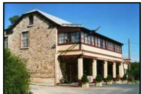
The ‘Bushranger Hotel’, formerly ‘Kimberley’s Commercial Hotel’
