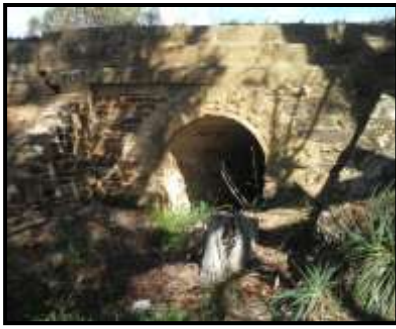
Culvert on Great South Road near Towrang Stockade
