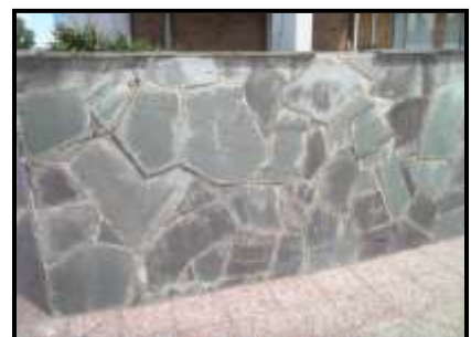
Façade of Chatsbury slate at motel in Auburn St. Goulburn
